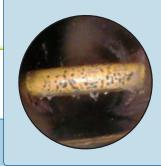
This photo, taken inside a sewer service line, shows a natural gas line that has penetrated the sewer service line.
