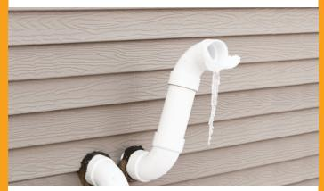
Sidewall vents act as a breathing device for heating systems. They take in fresh air and mix it with fuel to produce heat, while discharging exhaust fumes that can include carbon monoxide (CO).
